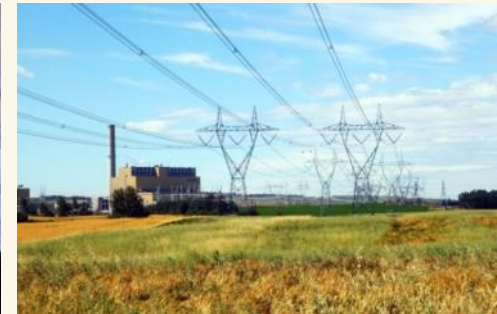
Electric Power Generation (EPG)
